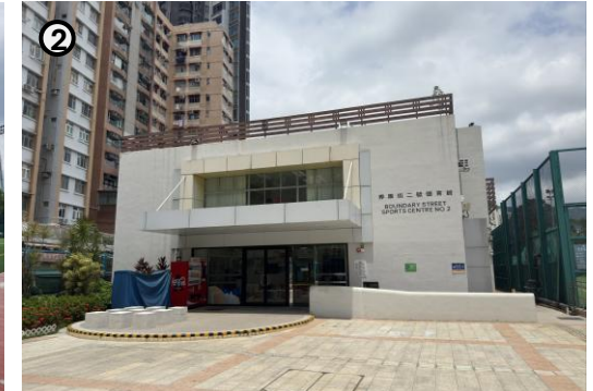
Boundary Street Sports Centre No.2
